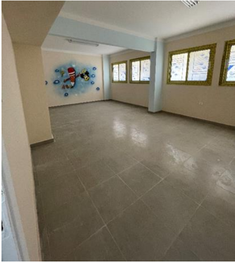
Figure 3: Classroom in Nursery
